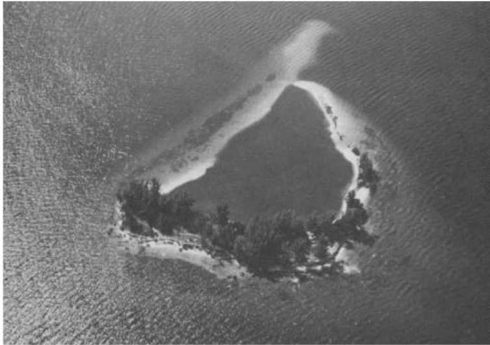
Figure 7-1. A dredged material island in Florida typical of those built in the U.S. Intracoastal Waterway
